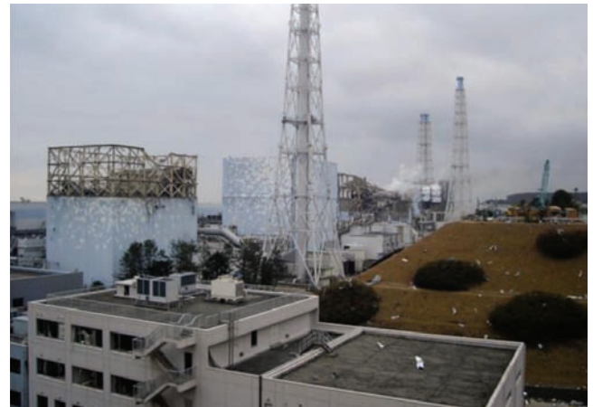
Unit 1 foreground, Unit 2 relatively undamaged structures, Units 3 and 4 background similar damage to Unit 1 (© TEPCO)
