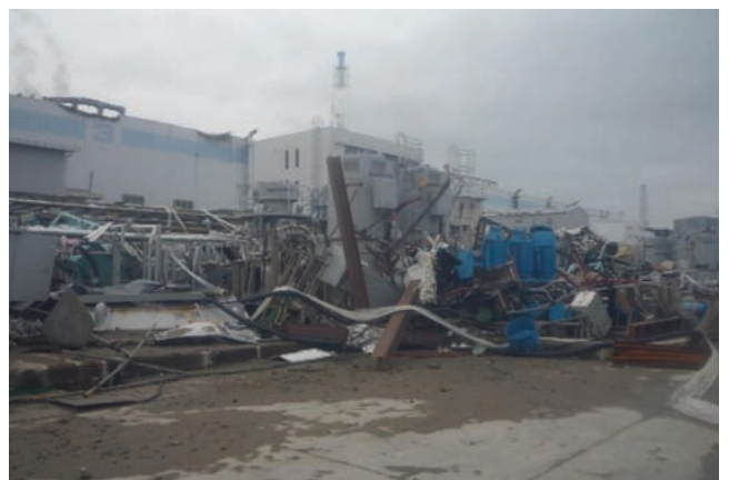
Damage at Fukushima Dai-ichi site following the tsunami (© TEPCO)
